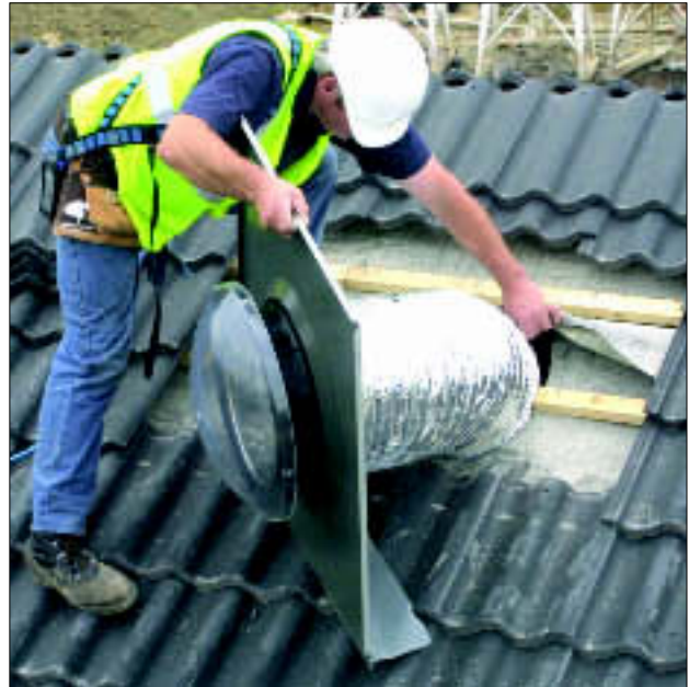
Figure 5 Installation of Sky Tunnel
