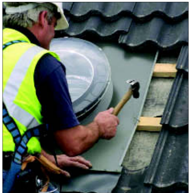
Figure 6 Installation of soaker tray
