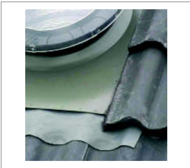
Figure 7 Lower tile lip detail
