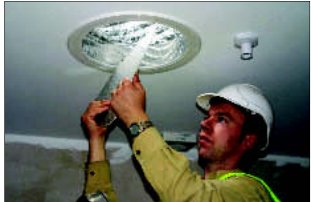
Figure 9 Installation of diffuser panel
